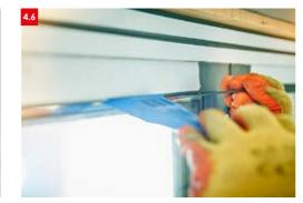
> 4.6 And the top corner which is diagonally opposite to the glass packing at the bottom.
