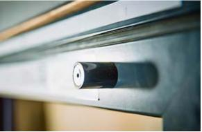
Check that the traffic door magnets have been fitted and that they align when in the open position.
