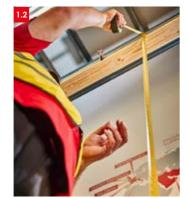
1.2 Check at least three height dimensions - both jambs and in the centre of the opening.
