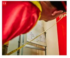
> 1.3 Check the opening for squareness by measuring the diagonals and check the frame for any damage.
