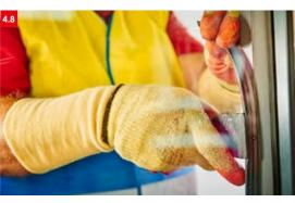
With weak soapy water (if required) fit the wedge gasket in one piece. Remember to force into the corners first and then loop from the centre towards the corners (if necessary snip the bottom of the gasket to facilitate ease of fitting at the corners) Ensure the wedge gasket is not stretched and
