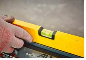
Recheck to ensure the cill is level and proceed to fix to substrate. Remember "check twice, fix once".
